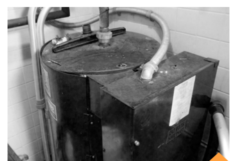
Rusted water boiler Mason Ridge Elementary
