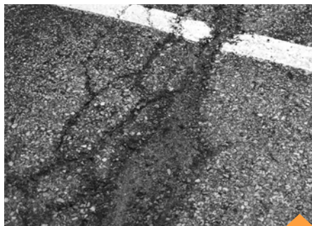
Fractured pavement McKelvey Elementary
