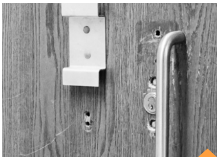
Damaged and aged door locks South Middle
