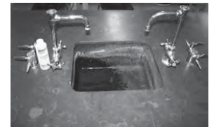
▶ Small, Corroded Sinks
