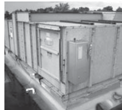
A battered HVAC unit at Northeast Middle
