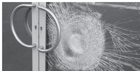
▲ Glass doesn't shatter when safety film is added to doors. An intruder is delayed.
