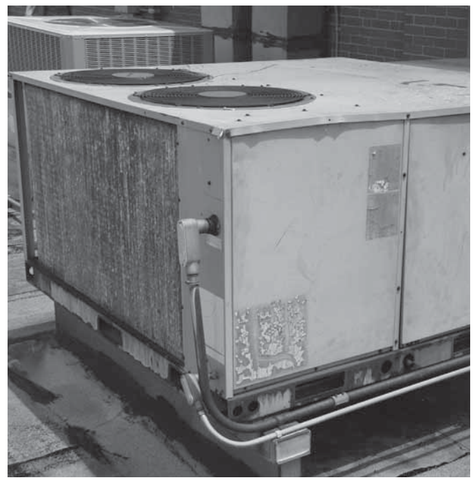
Mason Ridge HVAC unit
